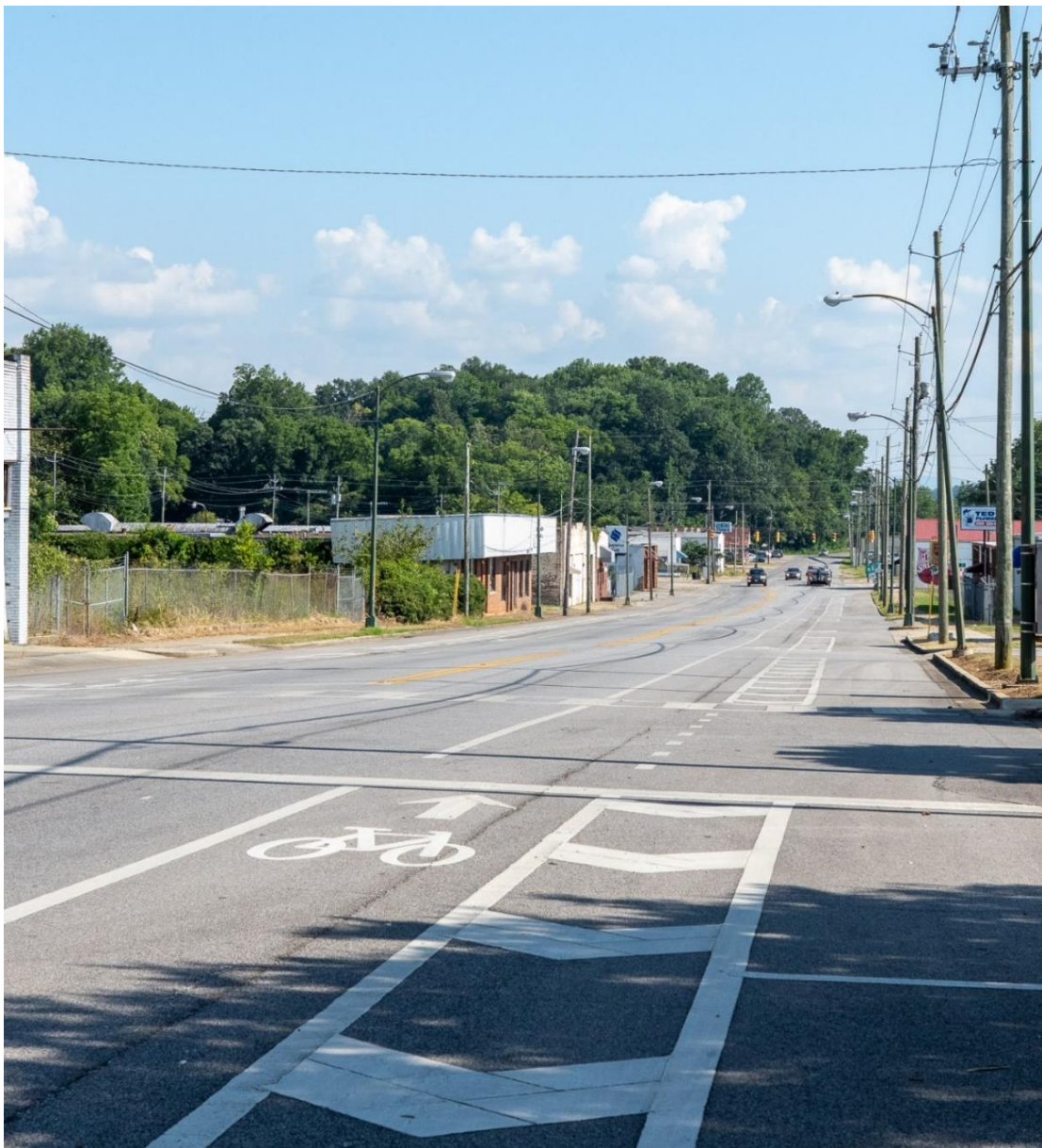
Figure 3-2: Example of Conventional Bike Lane along Noble Street in Anniston AL
