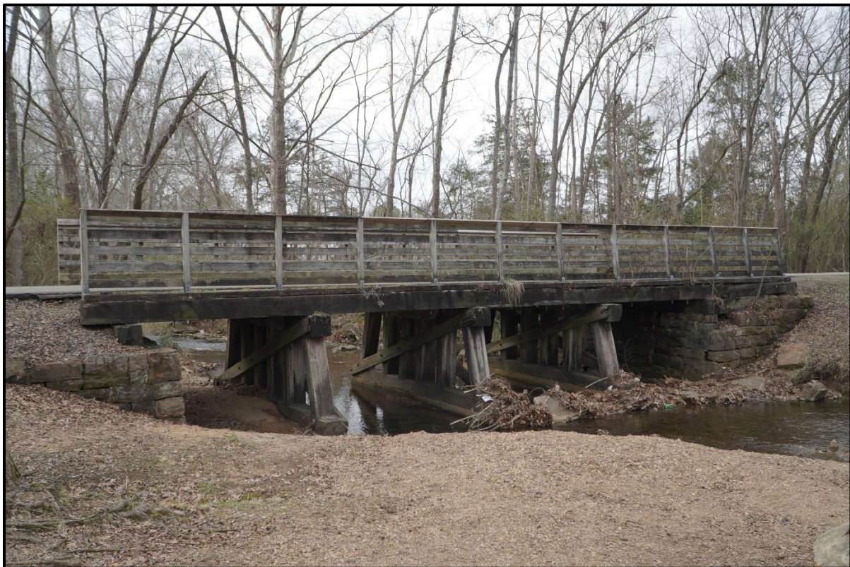
Figure 4-12: Retrofitted Railroad Trestle along Chief Ladiga Trail
