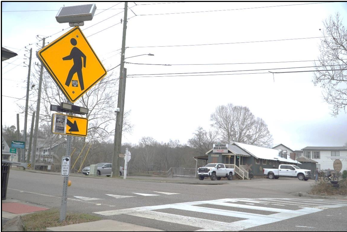
Figure 4-17: Example Active Warning Beacon
