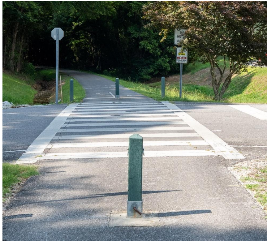
Figure 4-6: Example of Bollards along the Chief Ladiga Trail
