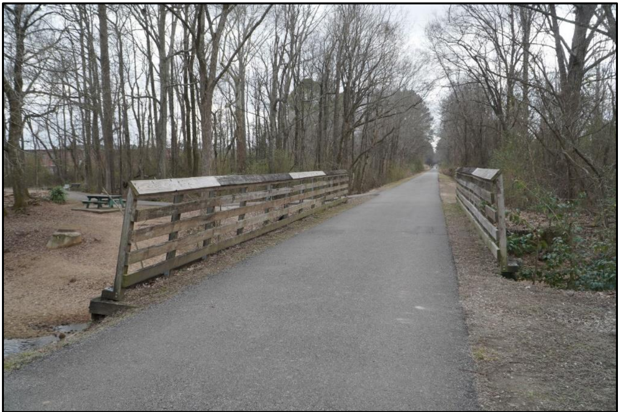
Figure 4-11: Example Bridge Approach along the Chief Ladiga Trail
